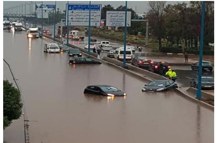
The main road from Casablanca-Rabat immersed in water during floods on 23 rd March 2016
