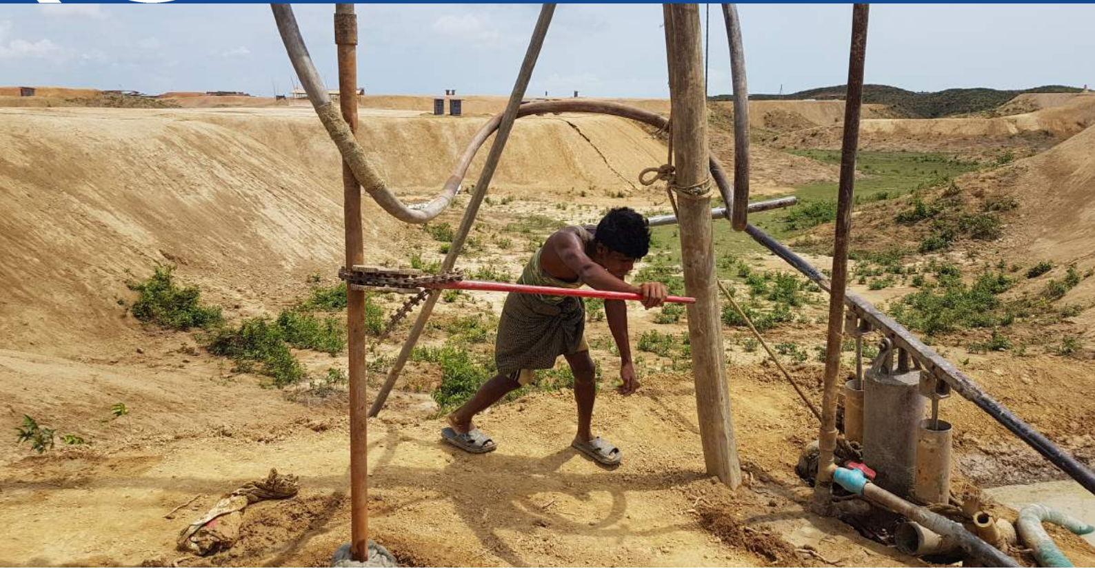
Manual drilling of a borehole in Cox's Bazar, Bangladesh. © A. Torres/IOM
