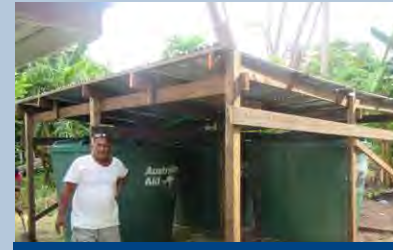
First rainwater collection unit in Piis-Paneu, Chuuk. Photo credit: IOM/Ambruce Mulo
