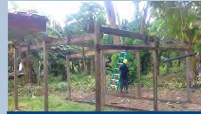
First rainwater collection unit in Piis-Paneu, Chuuk. Photo credit: IOM/Ambruce Mulo
