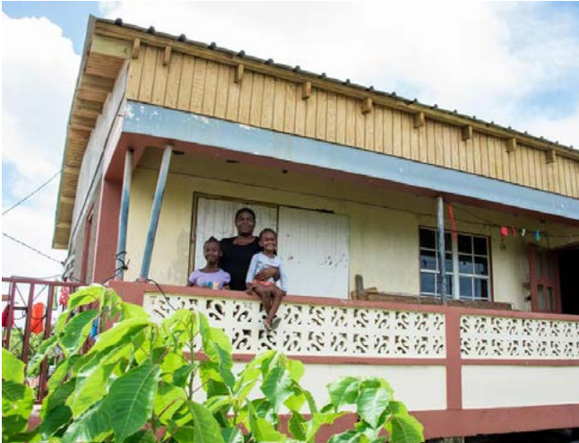
Houses repaired in Dominica © Sheldon Casimir / IOM 2018)
